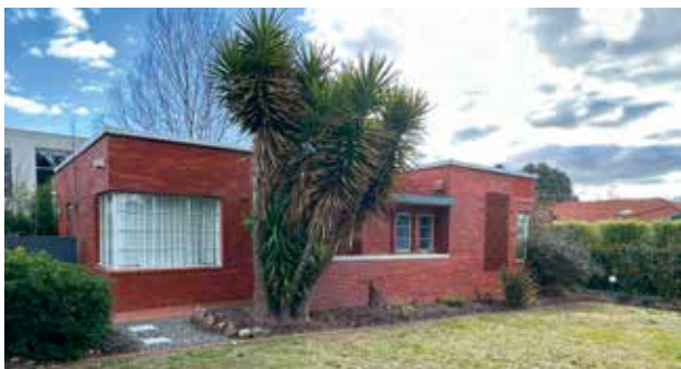
Whitley house, 107 Limestone Avenue [L Roberts]
