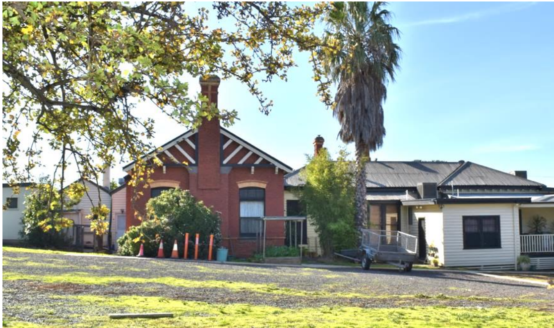
"Wilmerdale" in 2020 from a neighbouring property. Only the red brick room seen here survives. Image: supplied.
