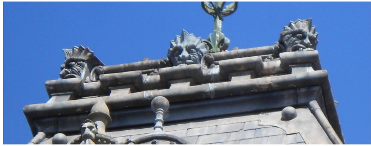
The watchers on the roof of the Bendigo Law Courts. Image: E Doling. The Bendigo Law Courts are on the Victorian Heritage Register VHR Number H1466.
