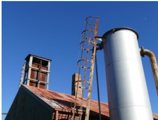
Bendigo former Gasworks, looking up. Photo: Bendigo Branch
