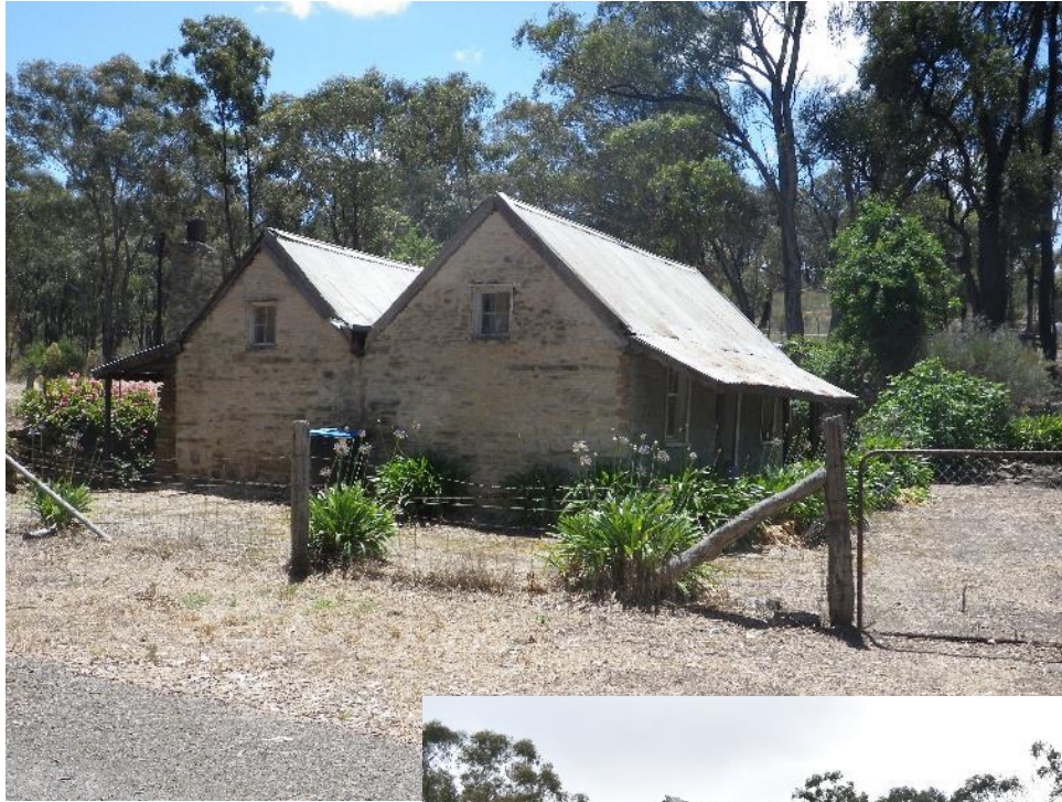
Figure 3: In 2012 the verandah and windows were intact. Photo: supplied
