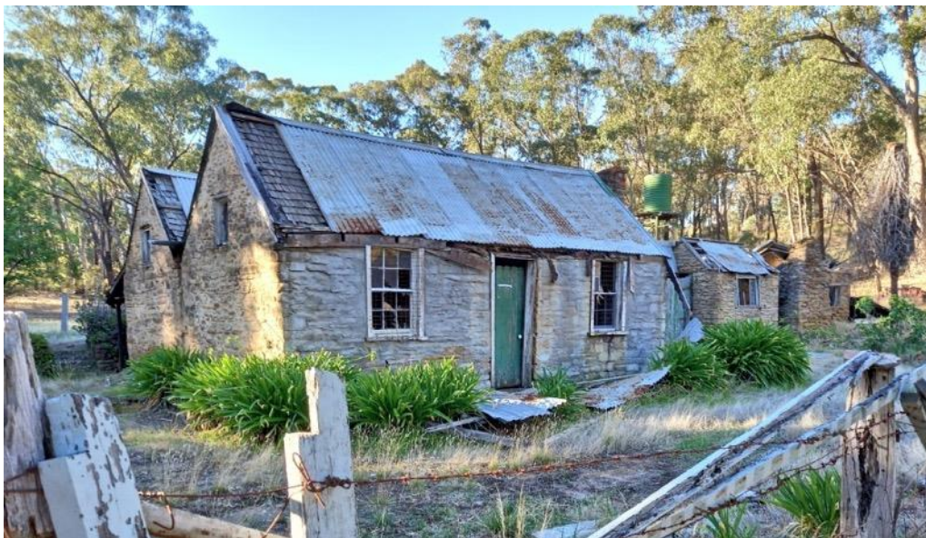
Figure 5: By April 2026 the verandah has completely collapsed, and iron is missing from the roof, exposing the shingles beneath and allowing water ingress. Photo: supplied
