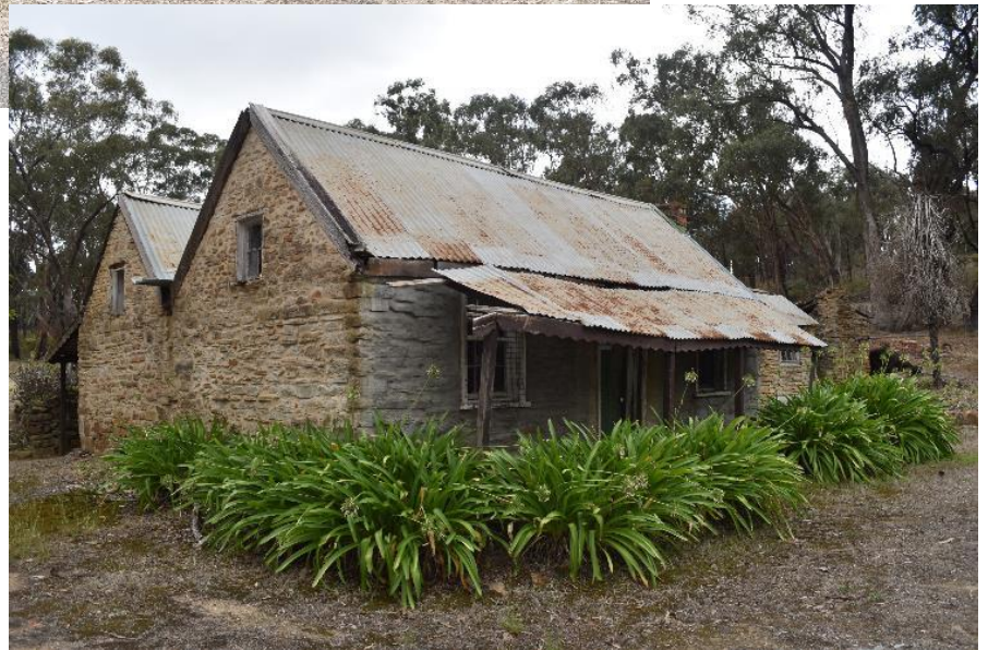
Figure 4: By 2022 all windows were smashed and the verandah was collapsing. Photo: supplied
