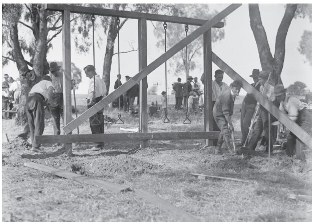
Corroboree Park playground working bee, 1926 [NAA: A3560, 840]
