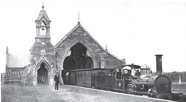
Rookwood Receiving Station No. 1, c. 1870s [All Saints Anglican Church, Ainslie]
