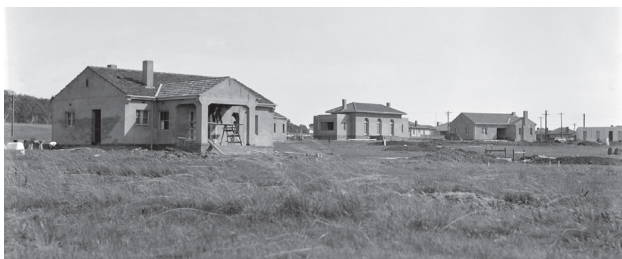
Alt Crescent houses under construction [NAA: A3560, 2377]
