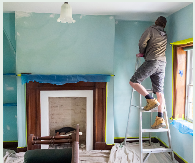
Conservation works at Hapers's Mansion. (Photography by Nick Nicholson)
