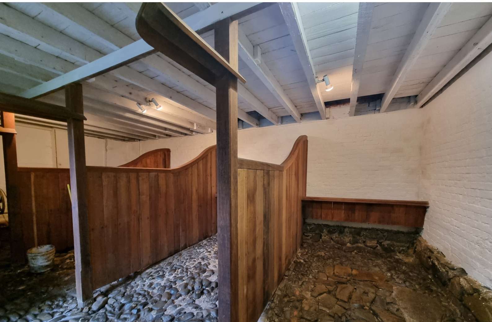
Franklin House Stables Following Completion of Renovation Works
