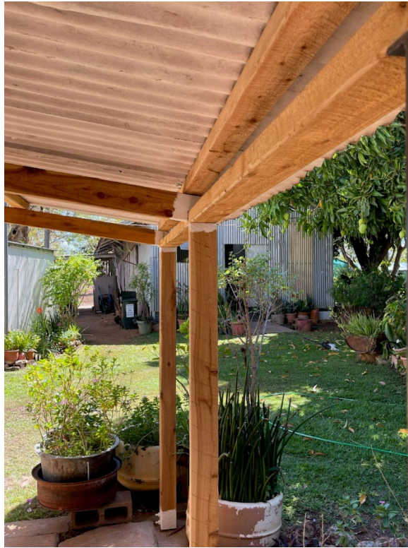
Replaced Cypress Pine roof beams 2024
