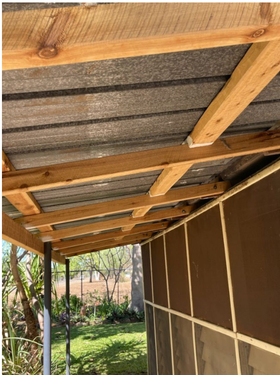
Replaced Cypress Pine roof beams 2024
