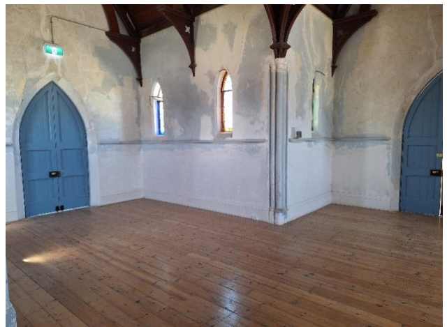
Before and after: left: Damaged render was removed and salt damp addressed. Right: Wall render and skirting reinstated and doors repaired and painted. Images: Gary Hill
