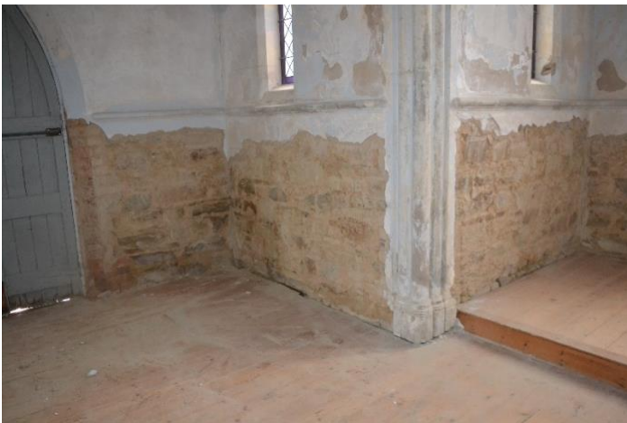
Before and after: left: Damaged render was removed and salt damp addressed. Right: Wall render and skirting reinstated and doors repaired and painted. Images: Gary Hill
