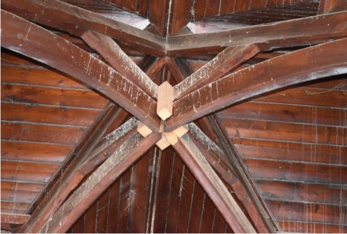
Above: before and after: left: Bird droppings on the roof trusses. Right: Roof timbers cleaned and walls repaired. Below: the North entrance before and after repairs. Images: Gary Hill
