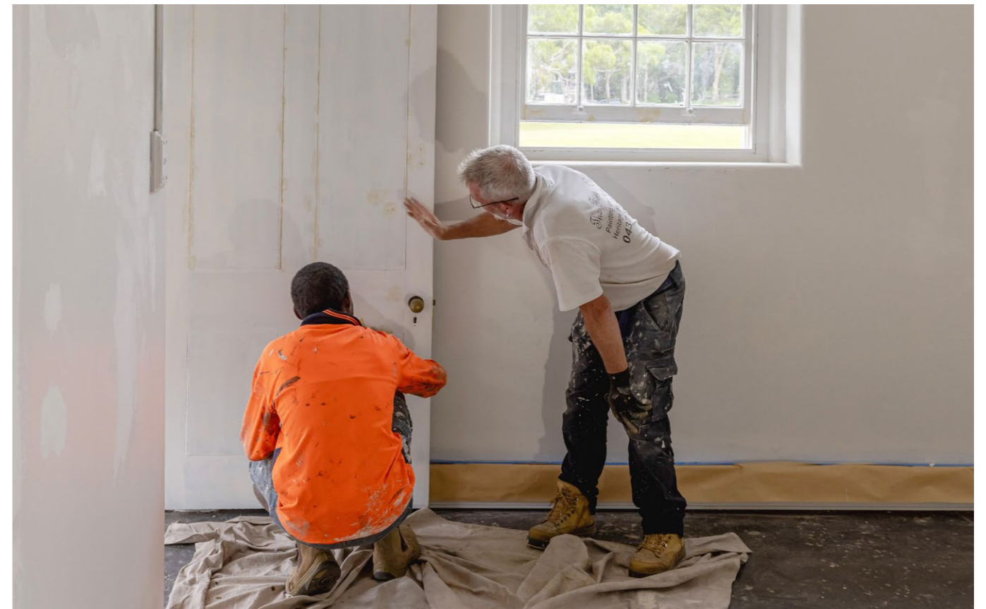
From top: The formal approach to Saumarez Homestead has been restored (photography Jarrad Stevenson); Conservation work at Old Government House (photography by Rick Stevens)
