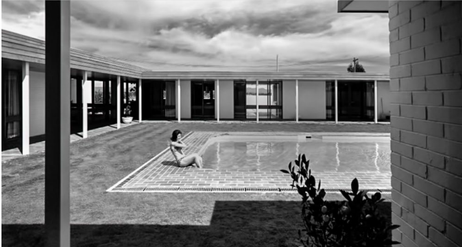
The Birch House, Yarralumla, by Noel Potter of Bunning and Madden - large expanses of glazing, overhang for shade cubiform overall shape. Source: Max Dupain and Associates Archives, all rights reserved.
