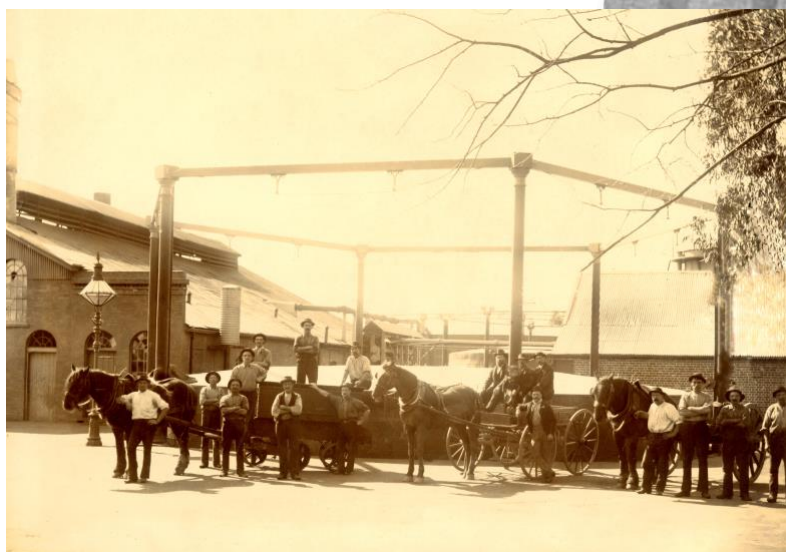
Below: Workers at Bendigo Gasworks about 1900. Wagon left has tram track wheels and the horse has skates on its shoes to run on the tracks smoothly and 'stay on track'. Image: Bendigo Historical Society
