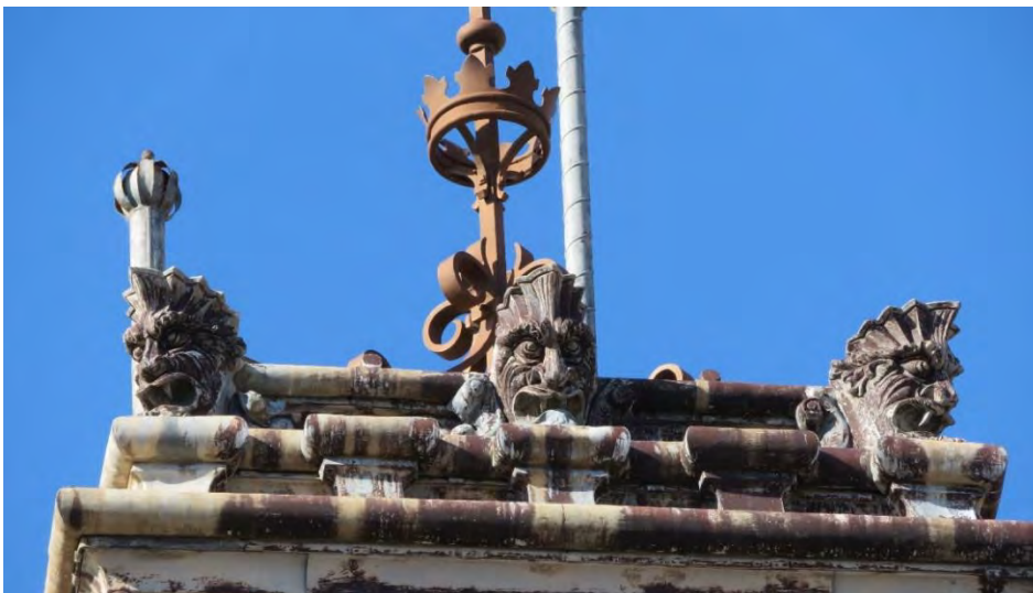
Figure 20 Mansard roofs to corner pavilions incorporate grotesque masks as acroteria and wrought iron finials; venting to the later waste water system is evident at the rear
