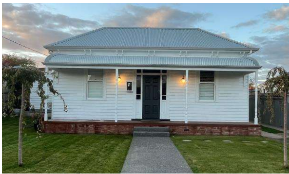
B0087, 618 Lydiard Street North, Soldiers Hill Replacement of corrugated galvanised iron roof, $4,000 awarded April 2022
