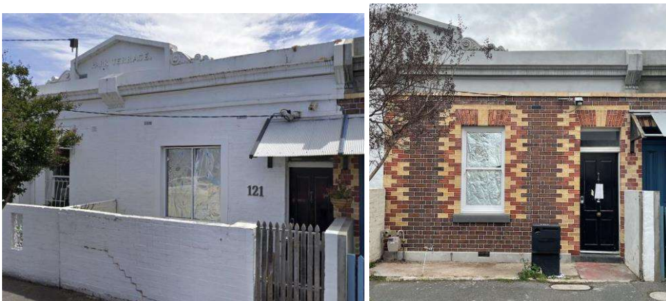
Y0096, 121 Park Street, Abbotsford Paint removal and reinstatement of original window, $6,000 awarded April 2021
