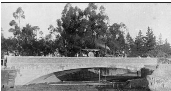
King's Bridge under test before failure
