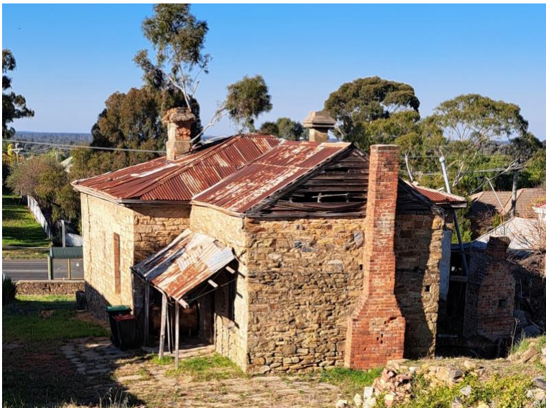
Rear view of a stone cottage on Eaglehawk Road, sent in by James Lerk. This illustrates the solidity and beauty of the stonework, but also how the cottage is at continual risk of damage with its rusted roofing, broken timbers in the gable and unstable brickwork of the chimney.
