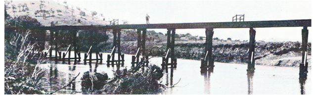
Timber trestle railway bridge looking upstream c.1920 [National Archives of Australia A3560, 230]
