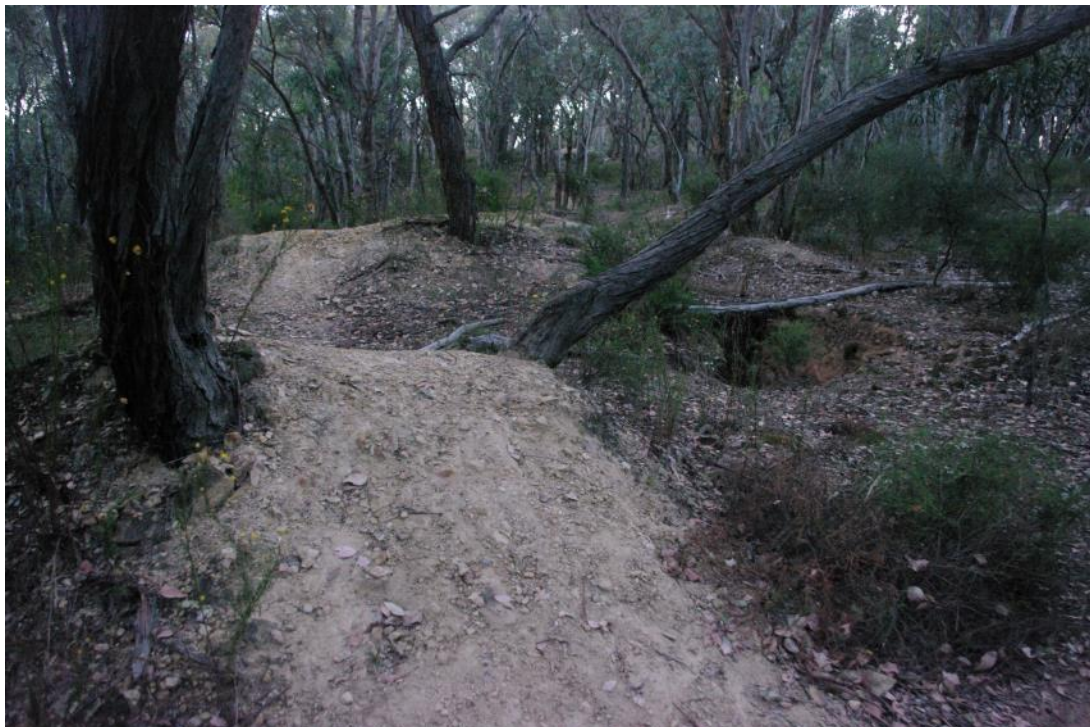
PHOTO 6. ILLEGAL MOUNTAIN BIKE TRACKS AND USE OVER HISTORIC MINING MULLOCK AND OTHER DISTURBANCE AND IMPACTS TO SITE
