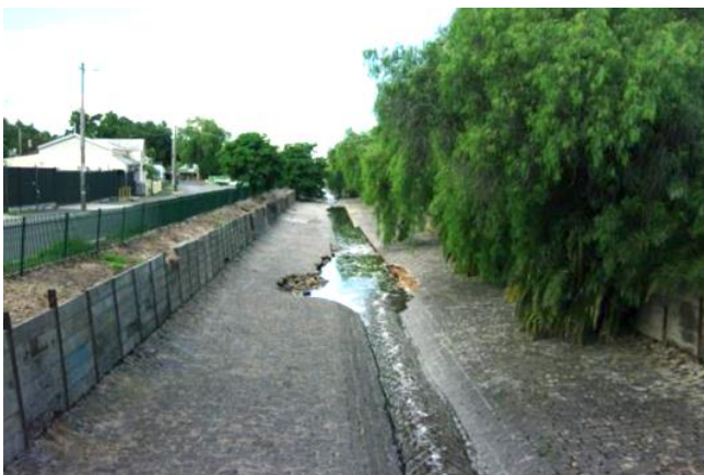
Bendigo creek bed bluestone blocks broken away and washed downstream. 9 Jan 2024. Image: Norm Stimson
