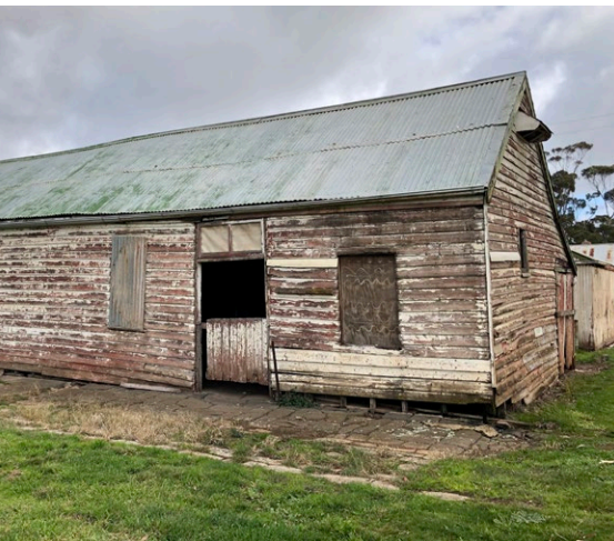
Before and after - Foundation supported stables restoration at Mooramong.
