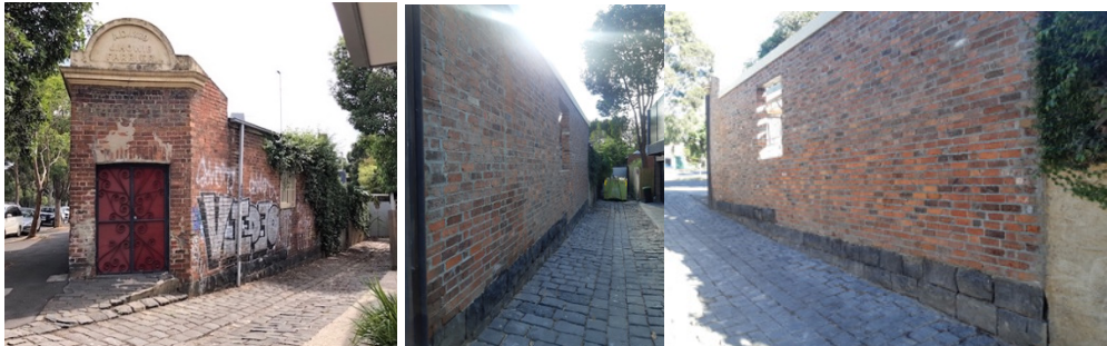
M0086 2A Curran St Nth Melbourne Re-building brick wall to match existing
