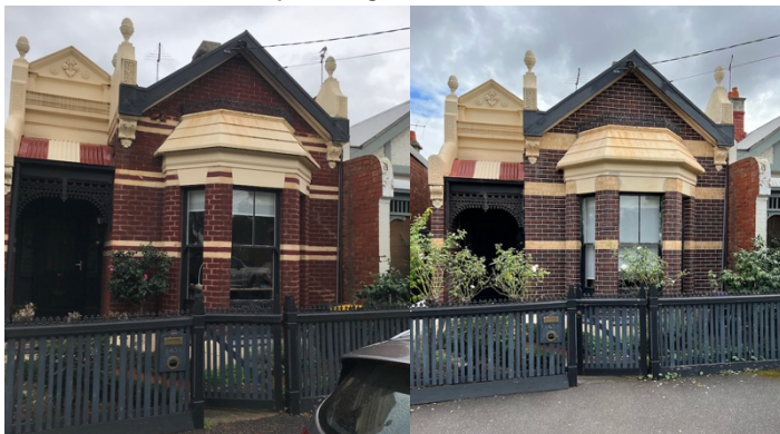
Y0087 43 Gordon St Clifton Hill Paint removal and repointing works
