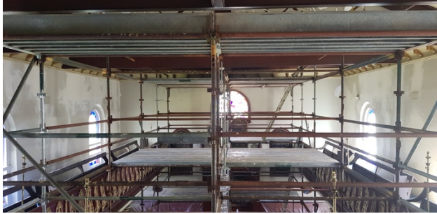
B0070 2 Barkly St Ballarat, Ballarat Synagogue Interior wall, joinery, ceiling restoration
