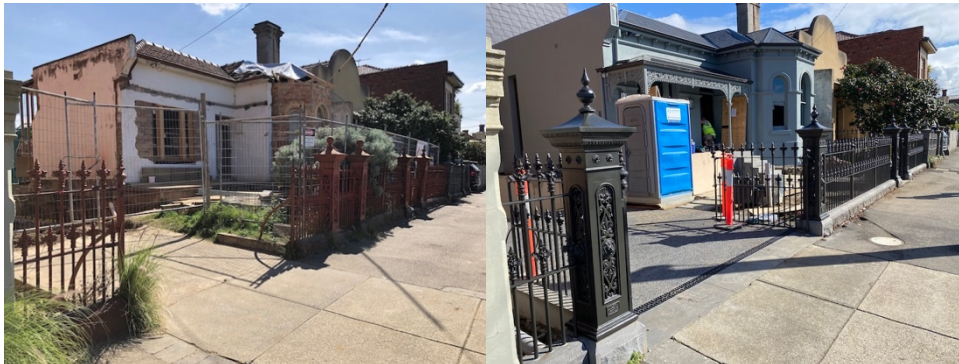
Y0081 417 Canning St Carlton Nth Restoration of the original cast iron fence
