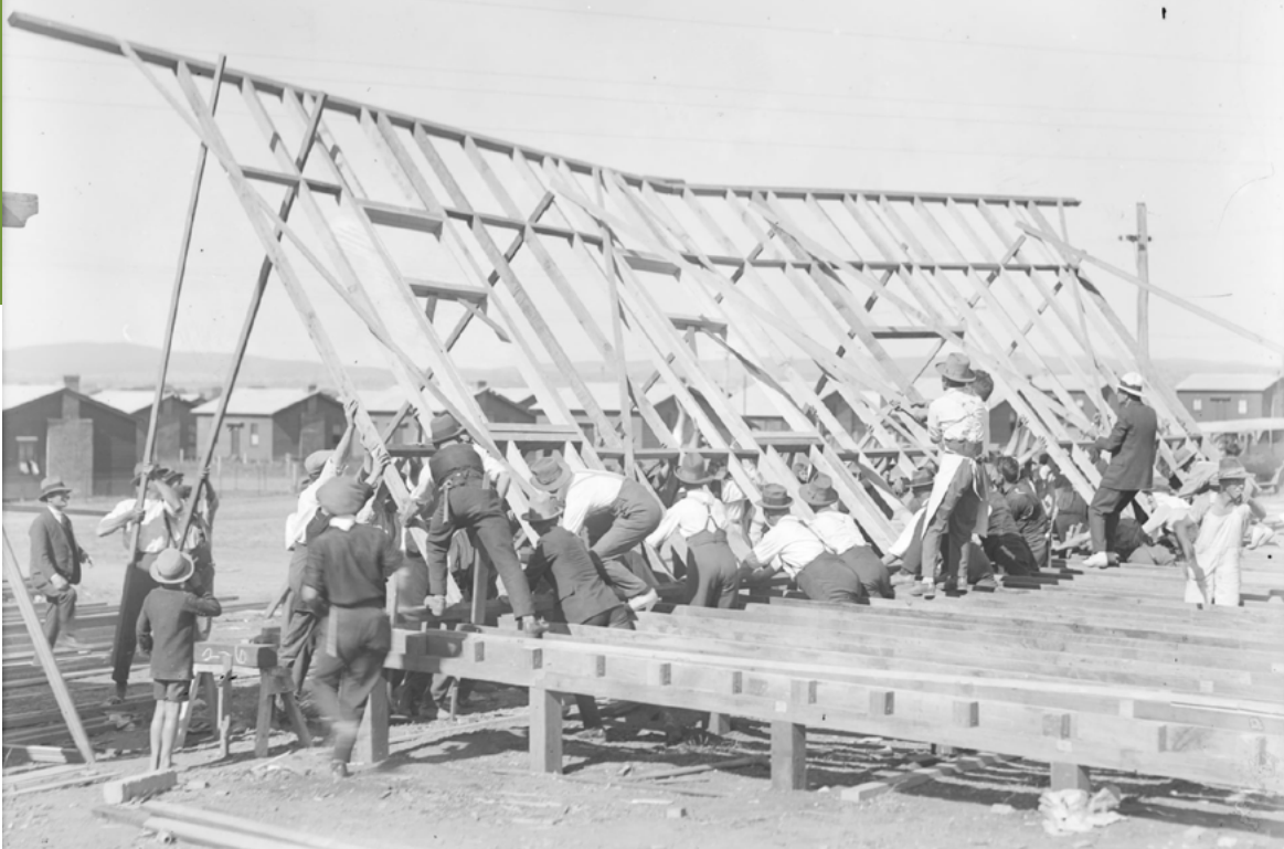
Raising a wall of the Causeway Hall, 1925 (Mildenhall Collection NAA: A3560, 785)
