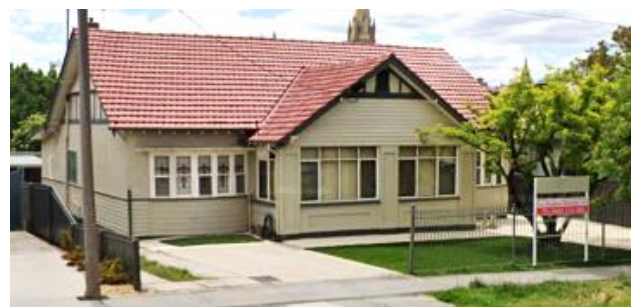
Example of a once residential dwelling in Hargreaves Street Bendigo, now used as commercial premises. Image: Google maps
