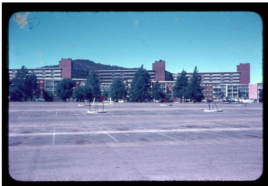
Allawah, Bega and Currong flats (1954). Designed by Richard Ure and Ian Slater, Commonwealth Department of Works.
