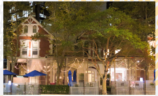
ABOVE: The Terrace Hotel on St George's Terrace is the former Bishop's Grove (G Pickering, National Trust of Western Australia)
