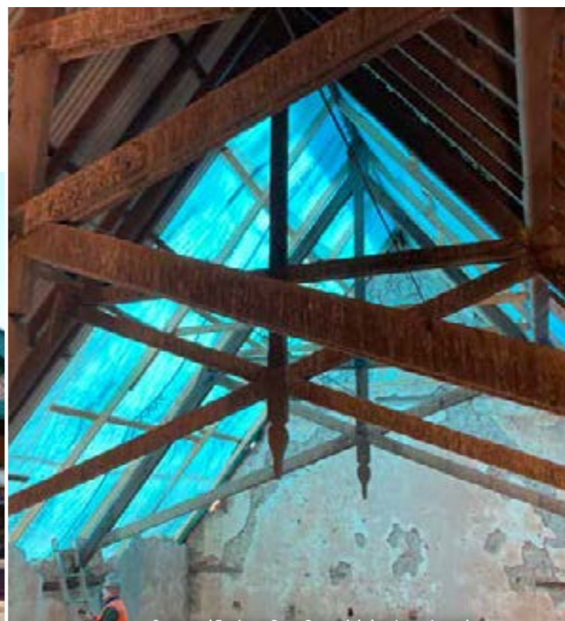
Structural Engineer Peter Baxendale has investigated structural damage caused when the Wesleyan Chapel roof was partially dislodged during cyclone Seroja in 2021. Photo: National Trust of Western Australia.
