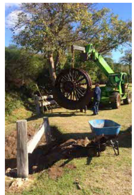
The water wheel being lifted back into its original location. Photo: Shelley Wightman.
