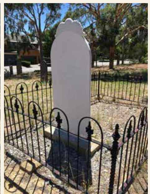
Barratt headstone showing marmorino finish at the back. Photo: NTWA.
