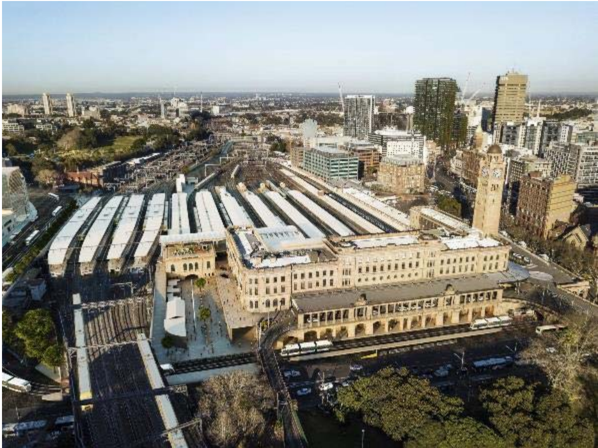
Central Station is a major defining element in the city, but also a significant barrier between parts of its immediate surrounds. (Source: Woods Bagot)
