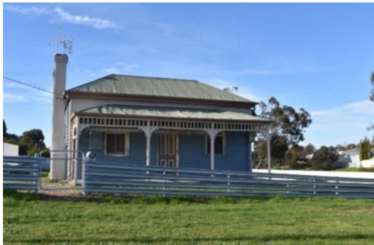
A basic weatherboard miner's cottage of the type promoted by The Bendigo Land and Building Society.
