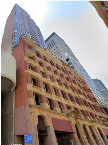
Museum Towers (267-277 Castlereagh Street)
