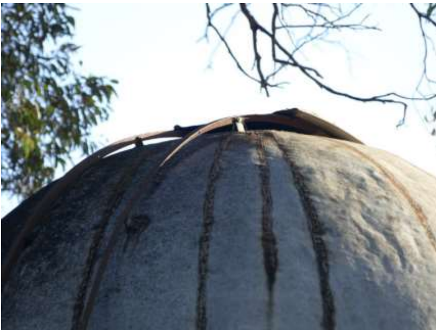
Figure 7: Observatory dome showing steel straps used in opening and closing the dome
