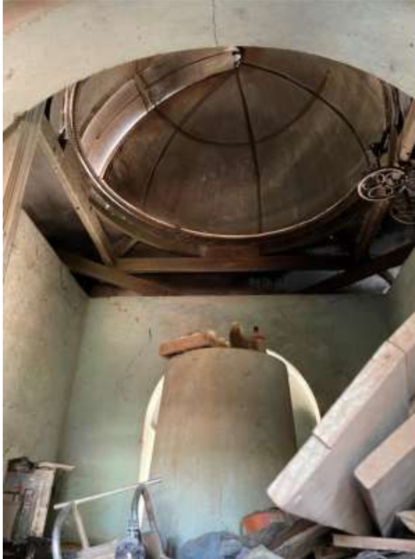
Figure 8: Interior of observatory showing the main dome, concrete telescope platform at centre and dome operating mechanism at top right
