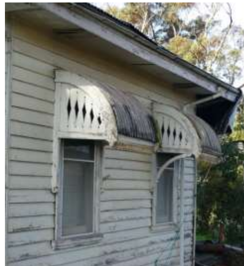
Figure 14: Original double hung sash windows and original window hoods
