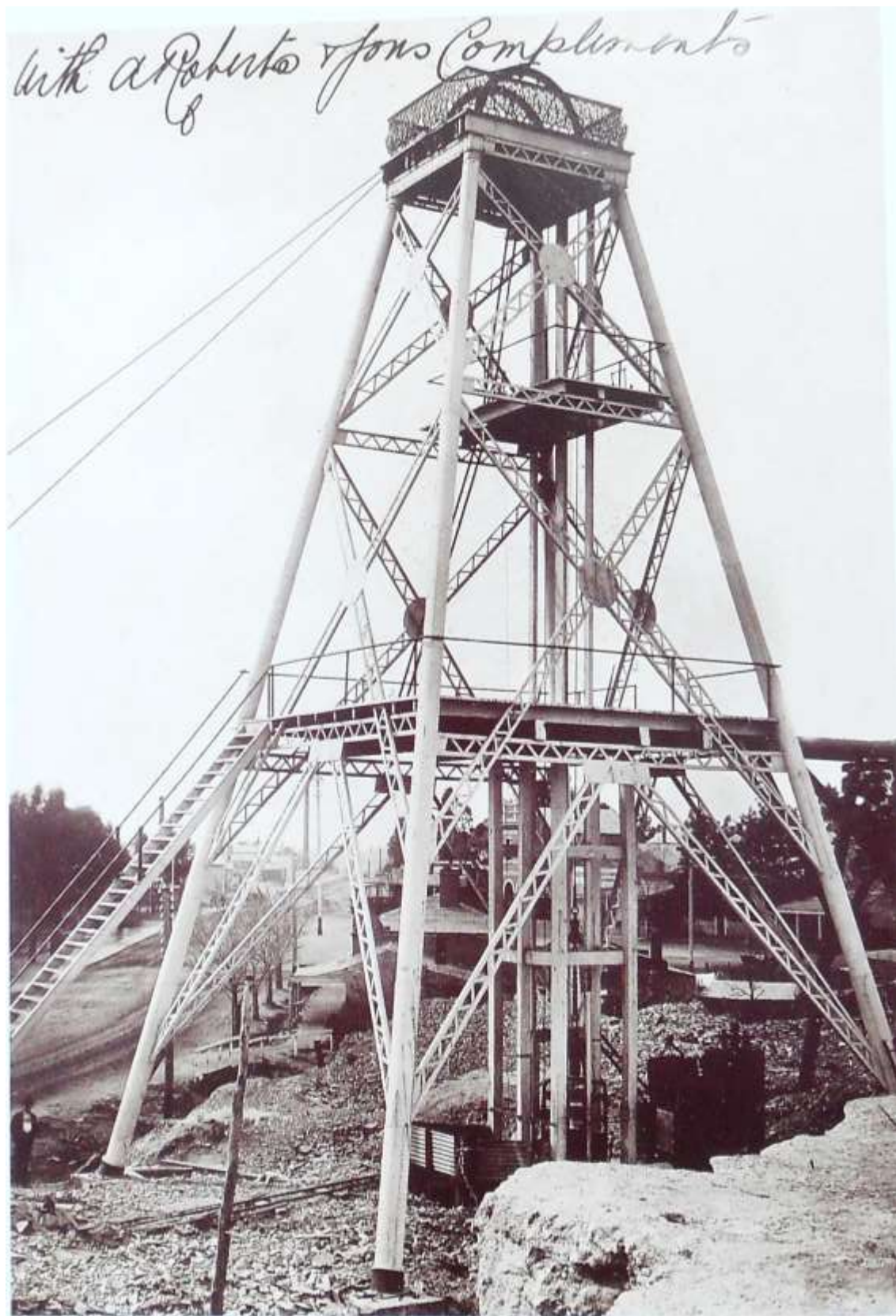
FIGURE 3: THE LITTLE 180 MINE POPPET HEAD, LOOKING TOWARDS IRONBARK TOWNSHIP C. 1897. ROBERTS AND SONS MANUFACTURED THE STRUCTURE. PHOTO W. H. ROBINSON FROM BENDIGO'S GOLD STORY, RALPH W. BIRRELL AND JAMES A. LERK.
