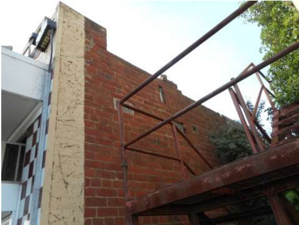
FIGURE 11: ORIGINAL SIDE WALL AND PARAPET OF THE BUTCHER'S SHOP. THE STEEL STAIRWAY GIVES ACCESS TO THE TOP FLOOR OF THE SHOP AND RESIDENCE NEXT DOOR.
