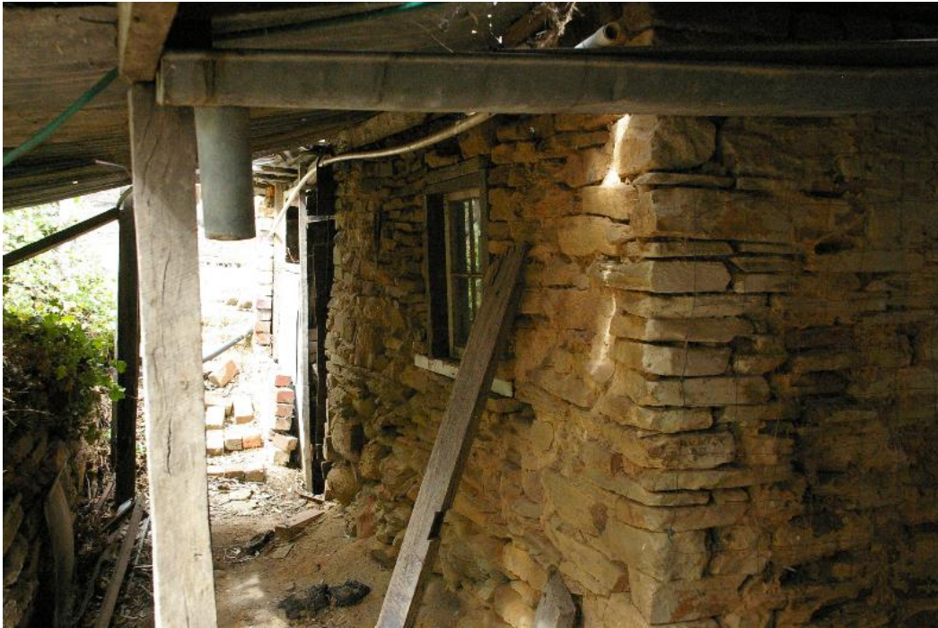
Figure 6: In 2012 the north side of rear bootmaker's workshop and verandah were still standing, although the wall was in need of repair. The verandah has since fallen down and the wall seen here has collapsed.
