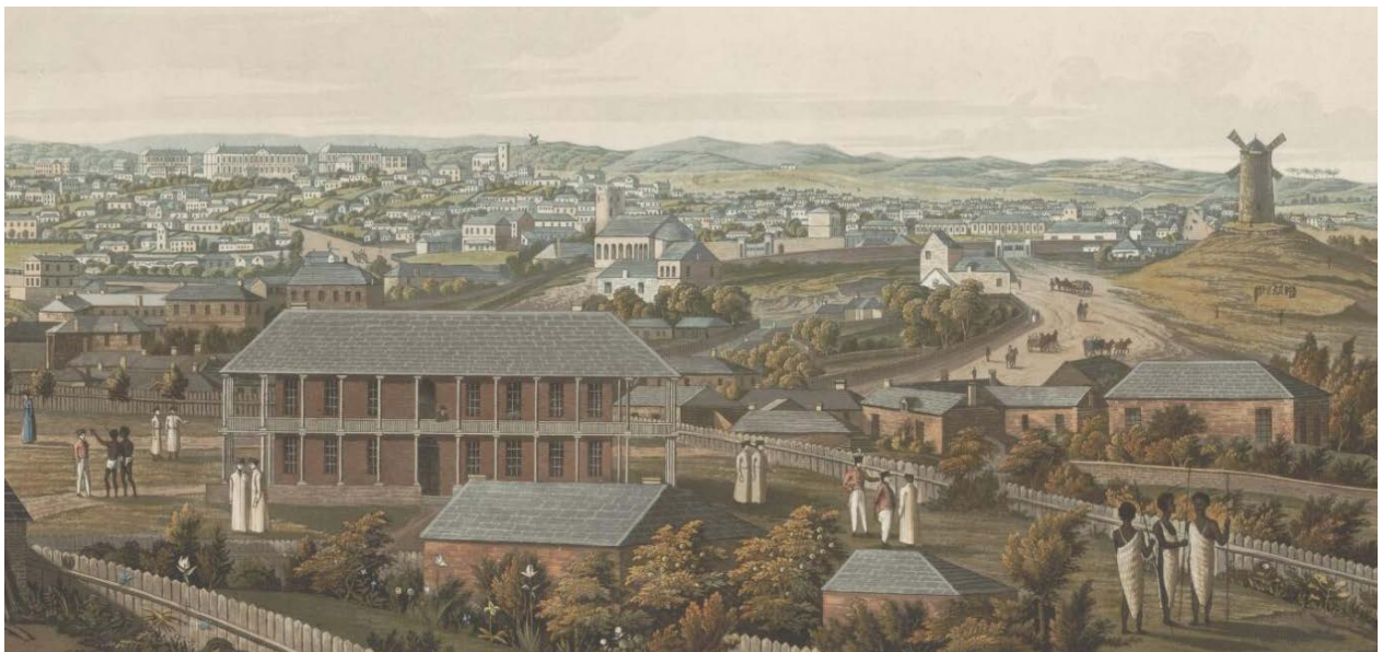
The town of Sydney in New South Wales , drawn by Major Taylor, 48 Regt. 1823. The main building in this image is the 1815 Military Hospital – now the National Trust Centre at Observatory Hill – and one of the earliest buildings in Australia. (Source: National Library of Australia)
