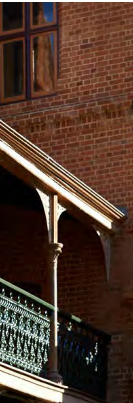
New cast iron balustrade bays to Woodbridge verandahs. Photo: National Trust
