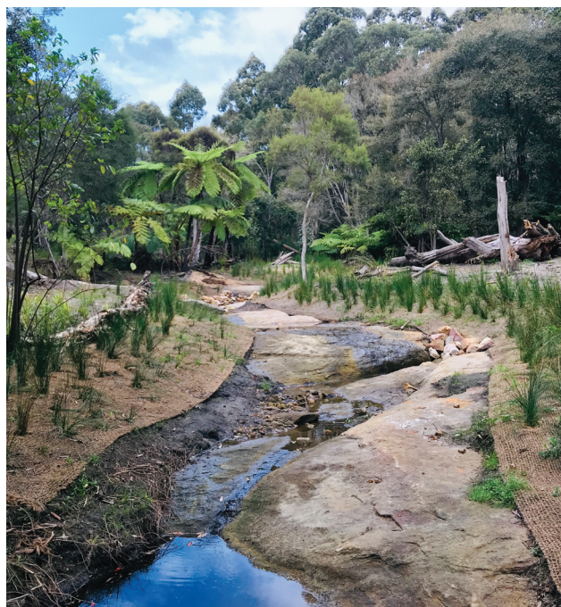
Rehabilitation works at Loftus Creek
