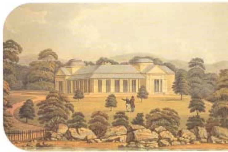
View of Captain Piper's Naval Villa at Eliza Point near Sydney, New South Wales by Joseph Lycett - published 1825. Courtesy Mitchell Library Australian Research Collection.
