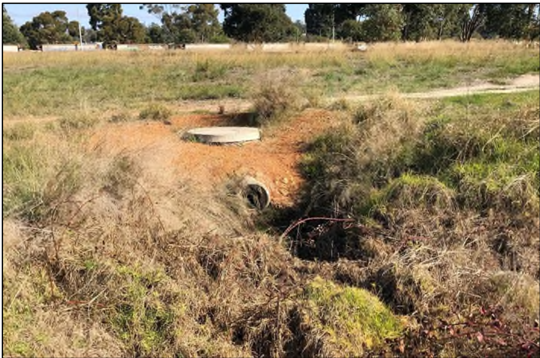
Plate 47: Underground drainage release point at ephemeral creek, located offsite.
