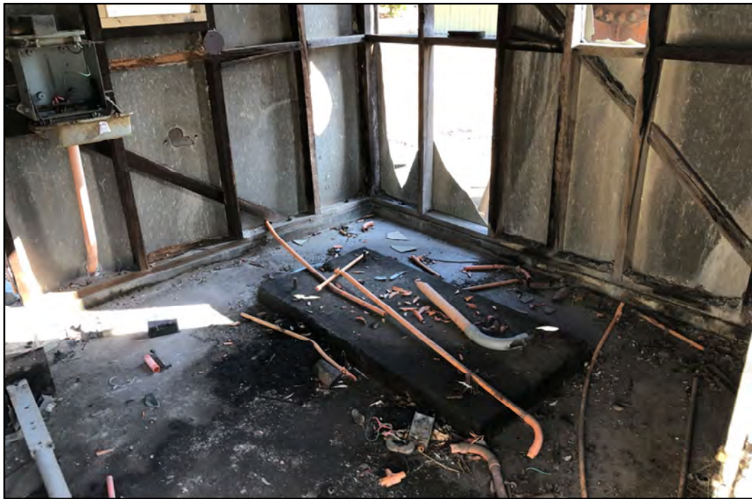
Plate 40: Inside the Compressor Shed. ACM fragments and black discolouration on the walls and concrete floor can be observed.
