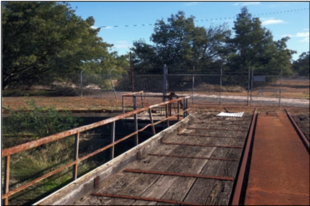
Plate 15: Turntable platform, looking north-west towards the manual operation pulley. The rusted steel and degraded decking are visible.
