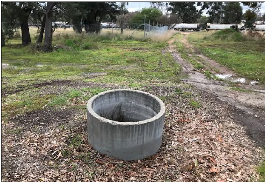
Plate 34: One of the soak wells observed in the eastern portion of Lot 561. The well was observed to sit atop the soil surface .
