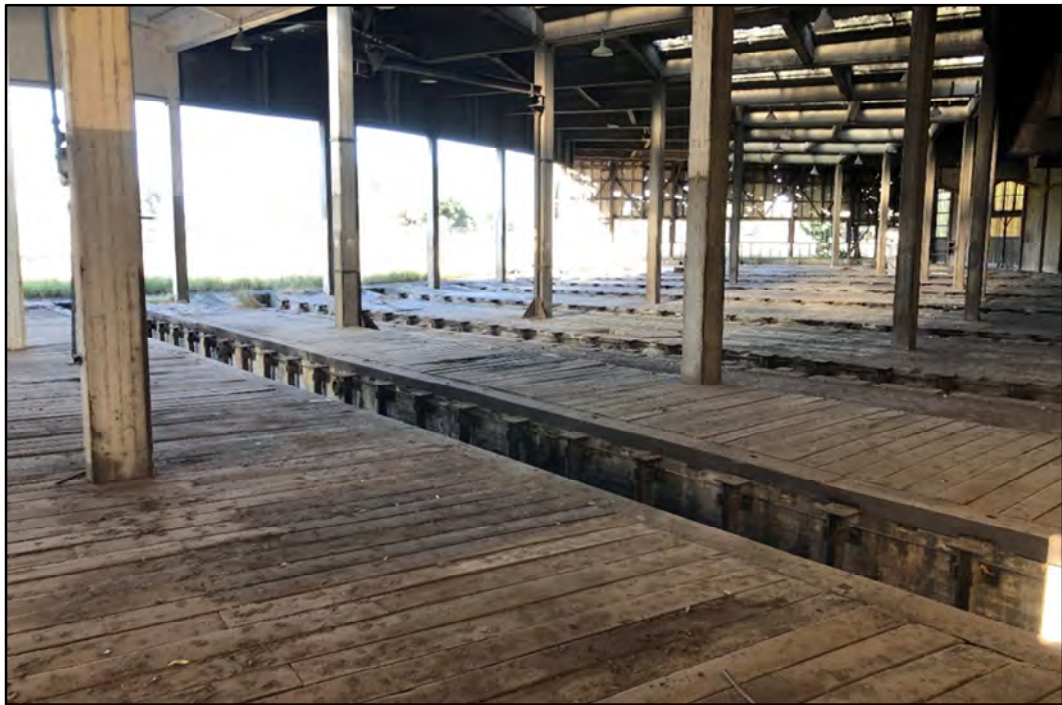
Plate 8: Minor staining on the timber floors within the Roundhouse.
