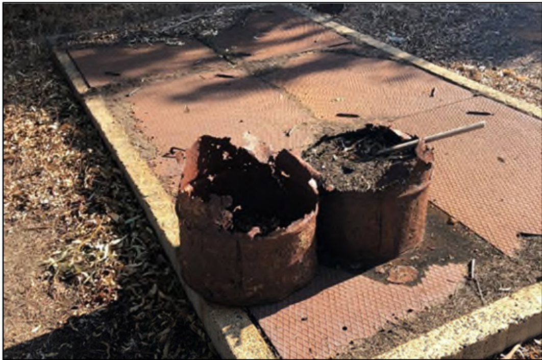
Plate 10: The two half drums on the triple interceptor trap. The drum on the right of the image contains the tar-like product, the other on the left was empty.
