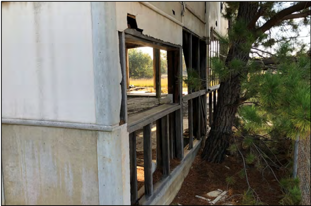
Plate 3: Damaged ACM cladding on the Roundhouse with ACM fragments visible on the surface soil.
