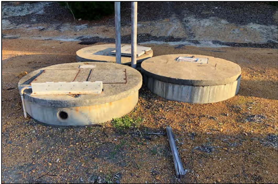
Plate 52: The three concrete lids, understood to be the septic tanks associated with the Aurizon Administration building.
