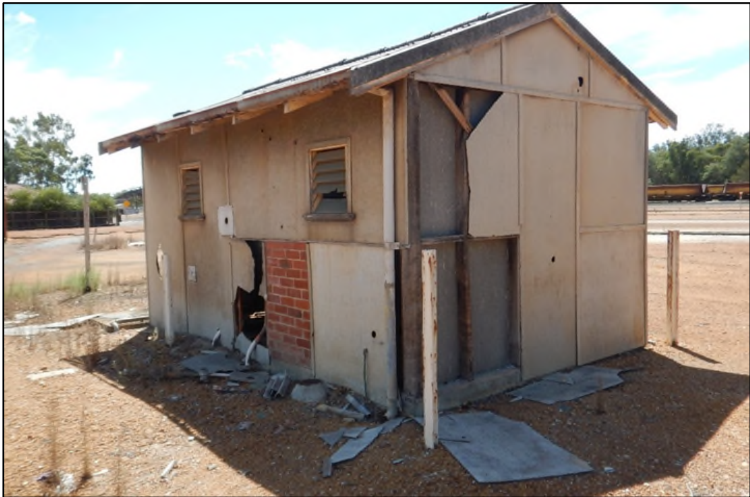
Plate 39: The damaged ACM cladding on the Compressor Shed. ACM fragments can be observed on the soil surface around the Shed.
