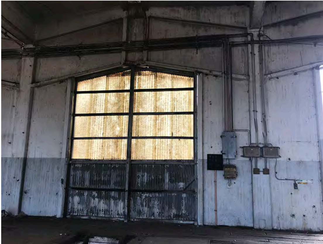
Photo 16 Detail view of opening in bay 3, with corrugated metal and plastic clad metal-framed gate.
