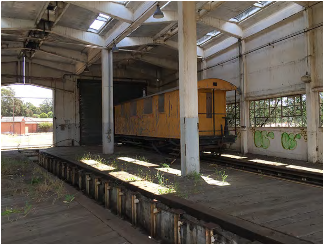
Photo 12 Looking north-west towards bay 1, showing train carriage. Note timber floor and painted concrete wall, columns and ceiling.
