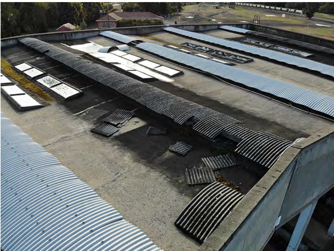
Photo 35 Detail view of roof showing asbestos sheeting, replacement metal sheeting and vegetation growing in valley, October 2018. (Image courtesy of Planwest)
