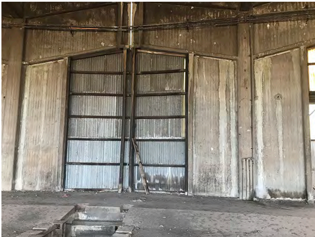
Photo 17 Detail view of opening in bay 8, with corrugated metal clad metal-framed gate.
