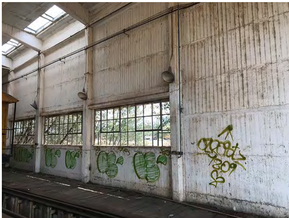
Photo 13 Looking north-west across bay 1 towards north end wall. Note off-form concrete wall, metal-framed glazing, skylights.
