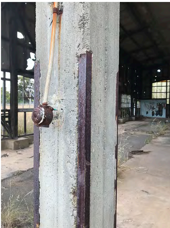
Photo 25 Detail view of missing cover to corner of column, showing typical damage to steel.
