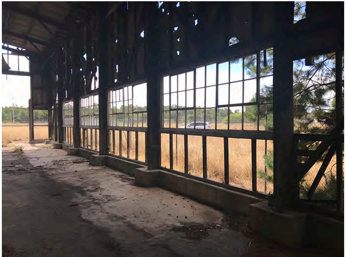
Photo 19 Looking towards east end wall showing framing and dilapidated asbestos cladding.
