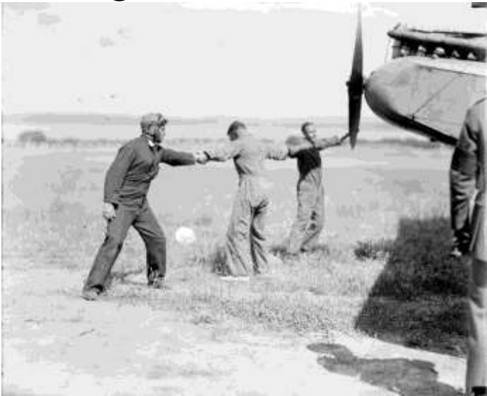
Observer and ground crew winding the propeller of a RAAF De Havilland DH9 at Canberra Aerodrome in 1925 (NAA A3560, 1519)
