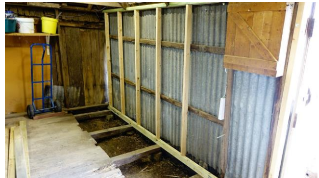
Above right: Earth excavated around bearers for ventilation; and the wall frame back onto bearers
