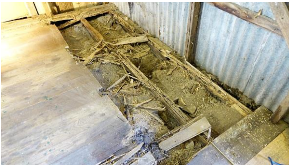
Above: Rotten floorboards but sound bearers
