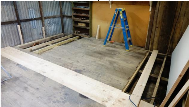
Below: Floor replacement in progress
