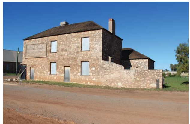
VIEW NORTH WEST
