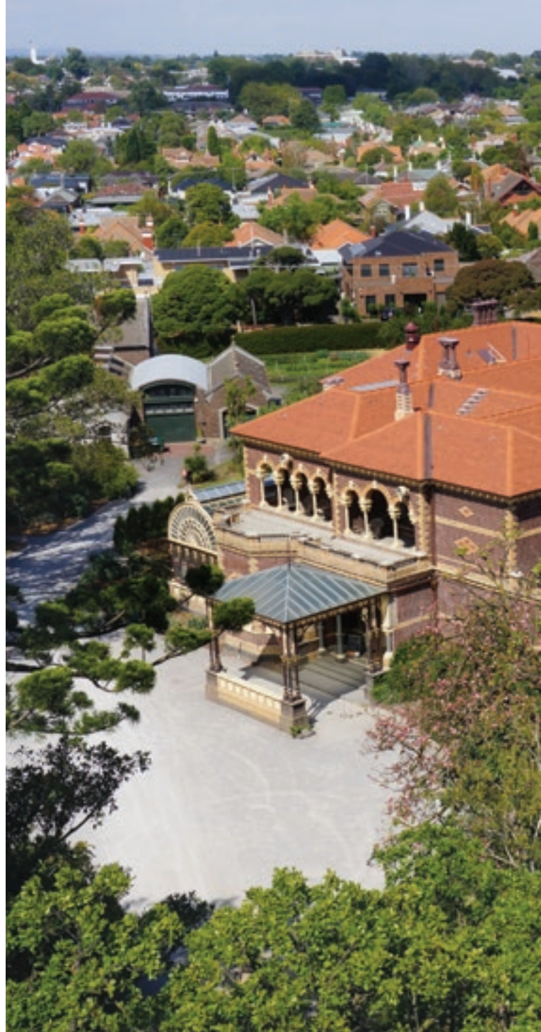
Custodianship of our Heritage: Ensuring sustainability of Rippon Lea through a reinstated roof and installation of photovoltaic panels.
