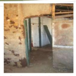
The collapsed dining room wall from rain from roof leaks, flooding and termite damage, the door arch reinstalled and timber beans reinstalled to brace walls replaced by water tank iron
