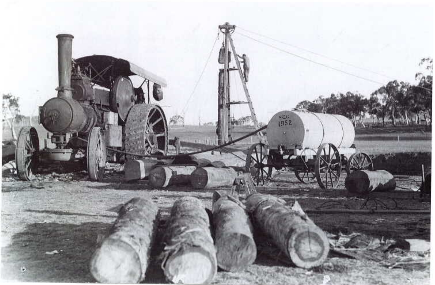
figure 5 (below): One of the 1925 Fowler engines operating a pile driving rig in the Woden Valley area. This engine is now exhibited at Lanyon.
