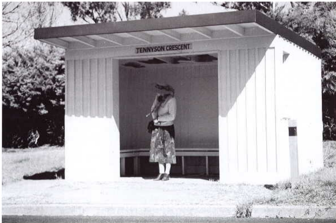
Class D bus shelter from 1944-45 on the corner of Empire Circuit and Tennyson Street. Its features include a sloping roofline, corrugated iron roofing, bench style timber seating, battened vertical timber with external strapwork, concrete slab floor, and two elongated side windows. photo: Peter Dowling
