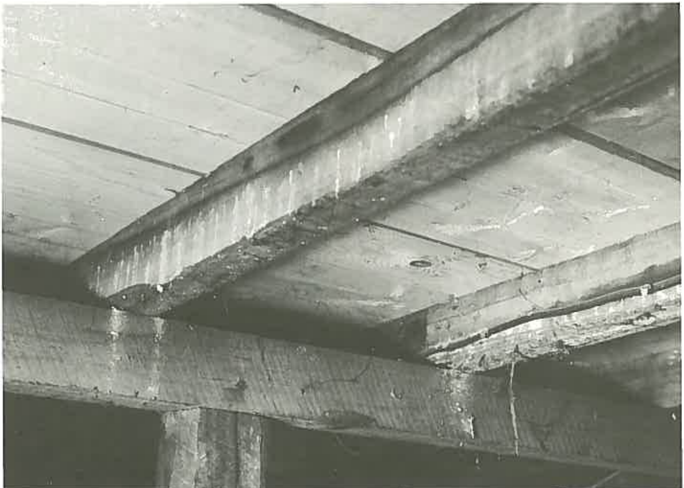
Lyctid attack in sapwood is readily recognised by the copious quantities of frass (borer dust) ejected from the infested wood.
