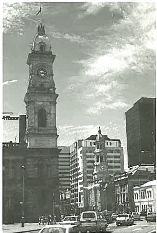
Plate 9: The tower of the Adelaide Town Hall in the centre of the photograph has been cleaned safely and effectively with a combination of water washing, bronze-wire brushing and chemical (ammonium bifluoride and hydrofluoric acid) treatment (on the more highly soiled parts). The tower of the GPO on the left has been cleaned by dry grinding which has left the surface of the sandstone and limestone damaged and spotty.
