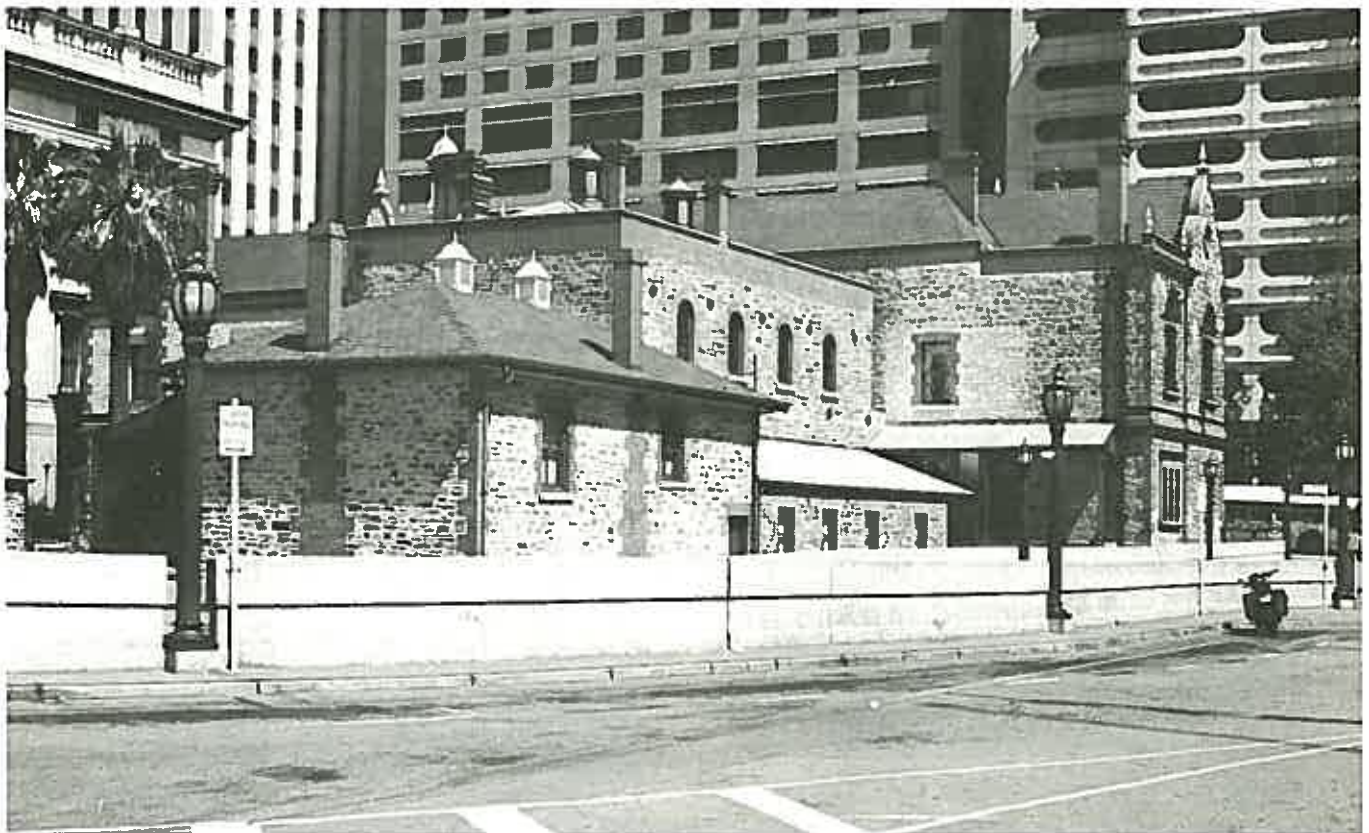
Plate 15: The degree to which cleaning is taken is a matter of judgement. The Old Legislative Council Building in Adelaide after 'restoration' in 1979-80 no longer looks 130 years old.
