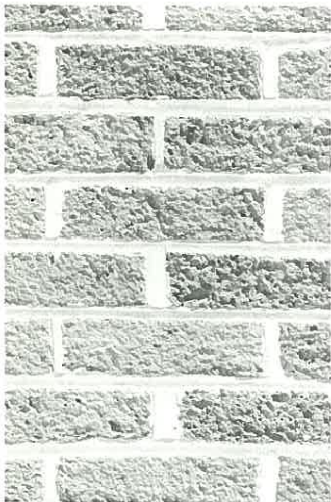
Plate 6: Dry sandblasted bricks in the 1863 Archer Street Police Station, Adelaide, have been deeply eroded. The original surface has been removed and the granular centre exposed.
