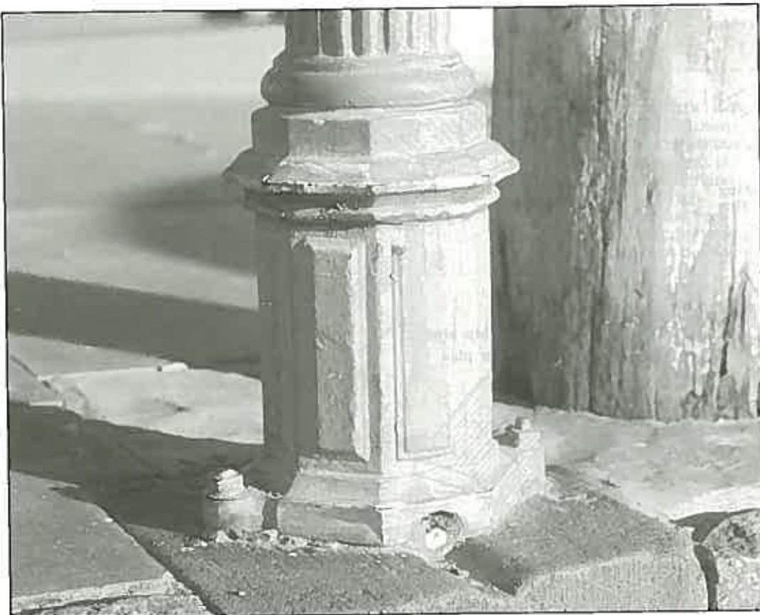
Base of a shop verandah column.
