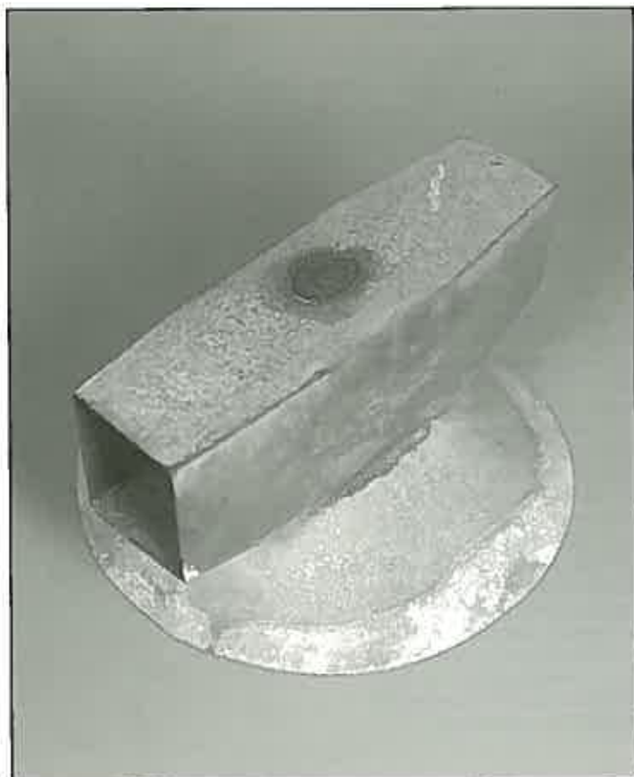
A patent ceiling ventilator found in the roof space of 'Glenfern', St. Kilda, designed to extract hot air fumes and water vapour from above a gas light fitting, and labelled as 'Murphy's Patent'. It was made by J. Murphy of Sandridge (Port Melbourne) in accordance with his patent of 1873, and dates from the installation of gas in the house in the 1870s.
