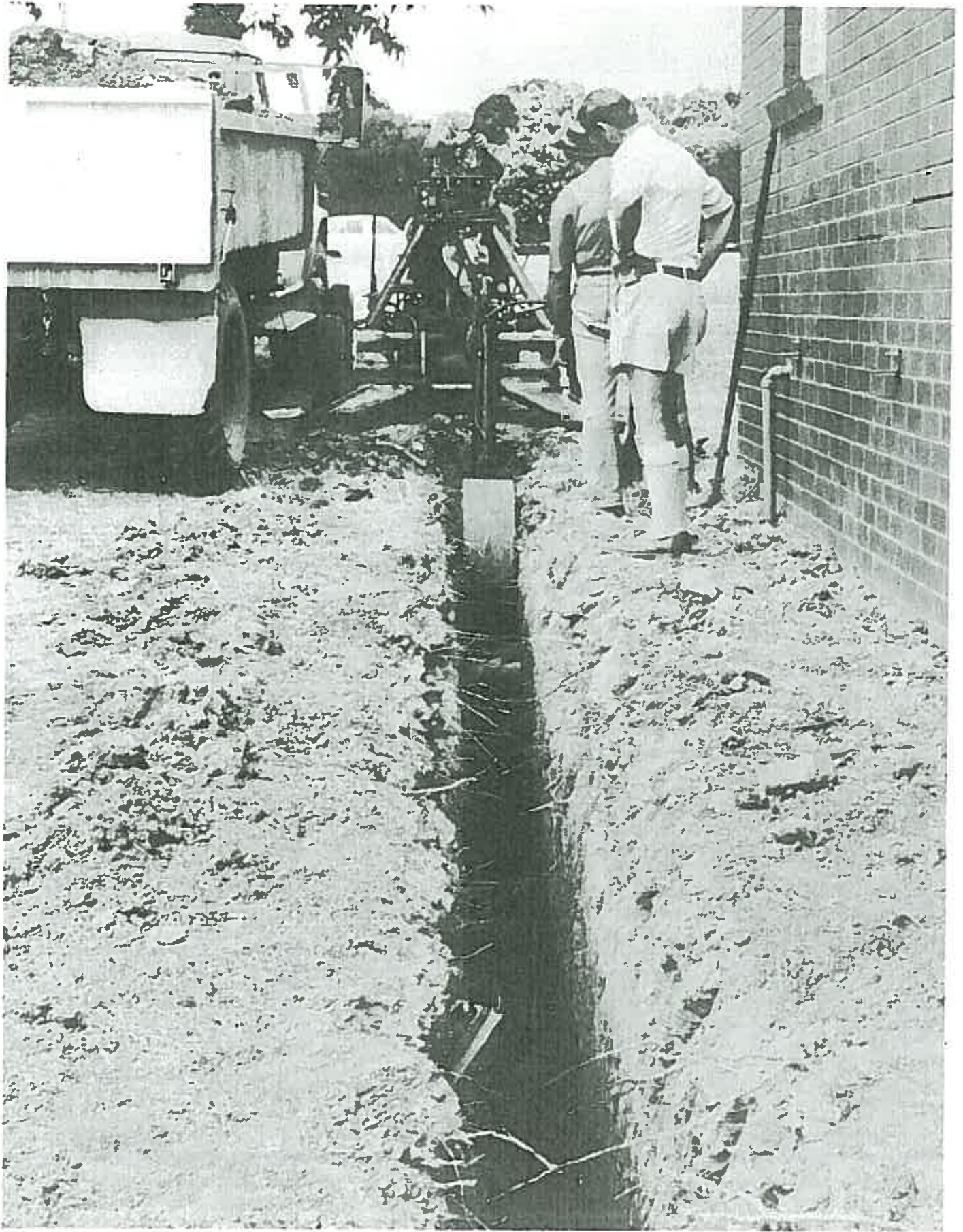
Figure 8b: Construction of a concrete cut-off wall.
